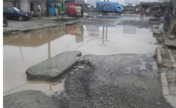
Figure 6b Bad road
